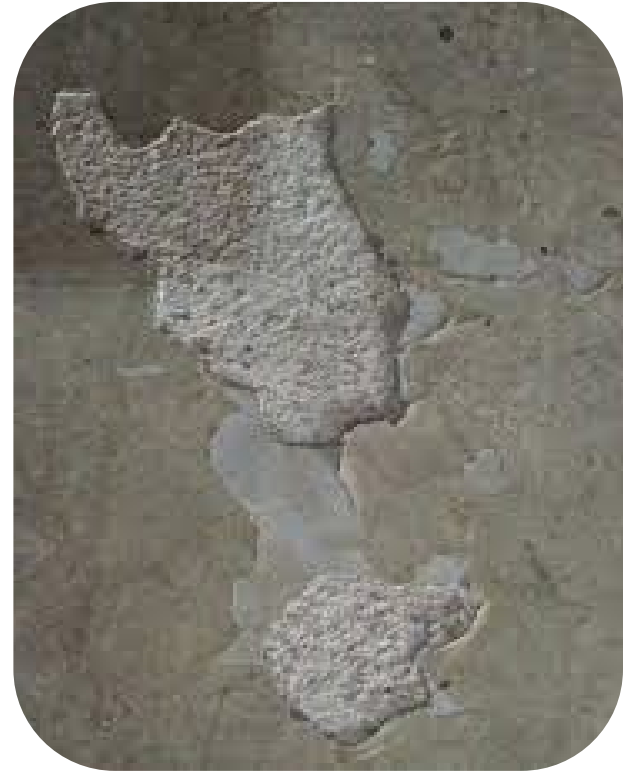
Delamination/rust
