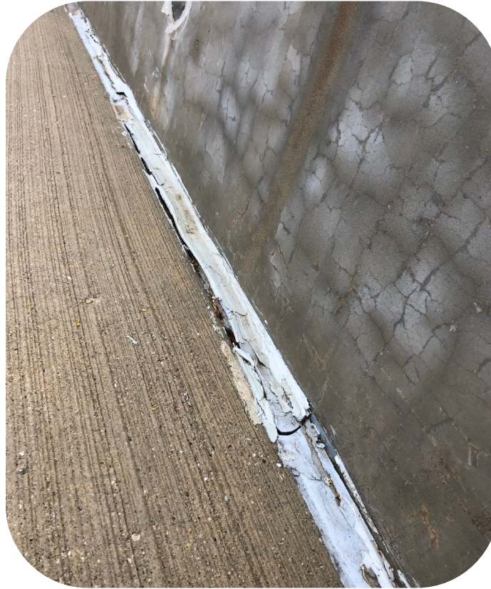
Deteriorated Sealant
