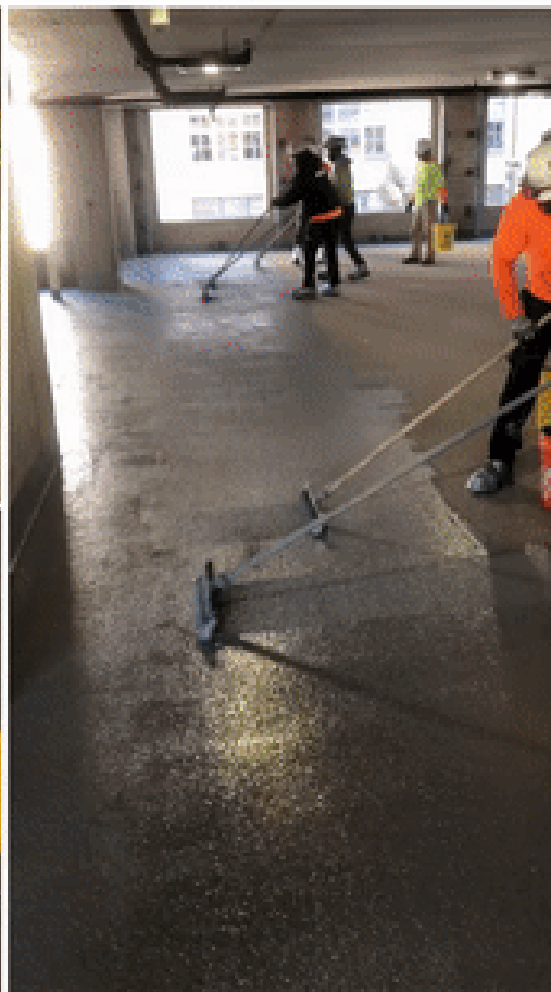
Western's DC branch installing a final coat of deck coating in downtown Baltimore steps from Camden Yards.
