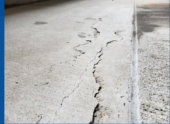
Reinforcement placed too close to the surface of the topping slab, resulting in the top surface failing due to rust jacking
