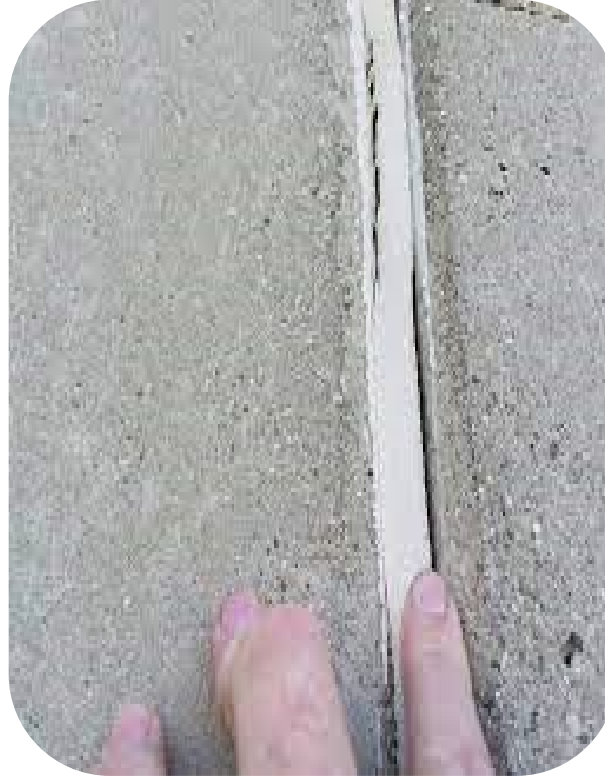
Typical Sealant Joint approx. $6/LF to replace
