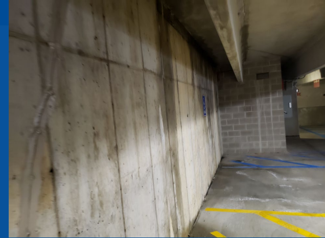
Water infiltration in a below grade parking level due to lack of water proofing
