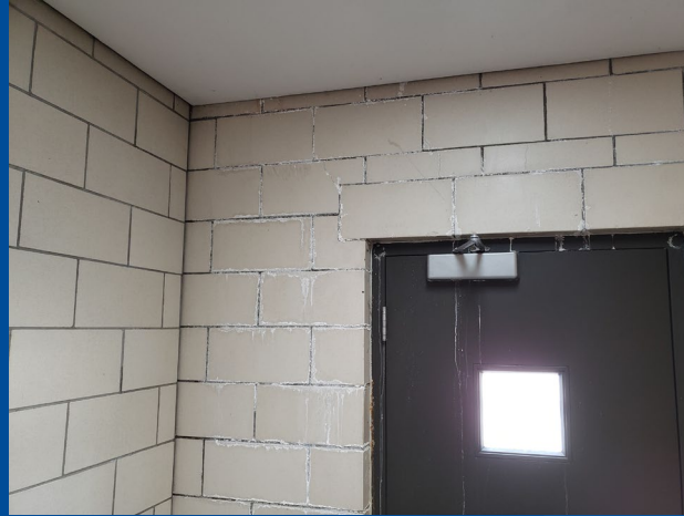
Water infiltration due to failed roofing system
