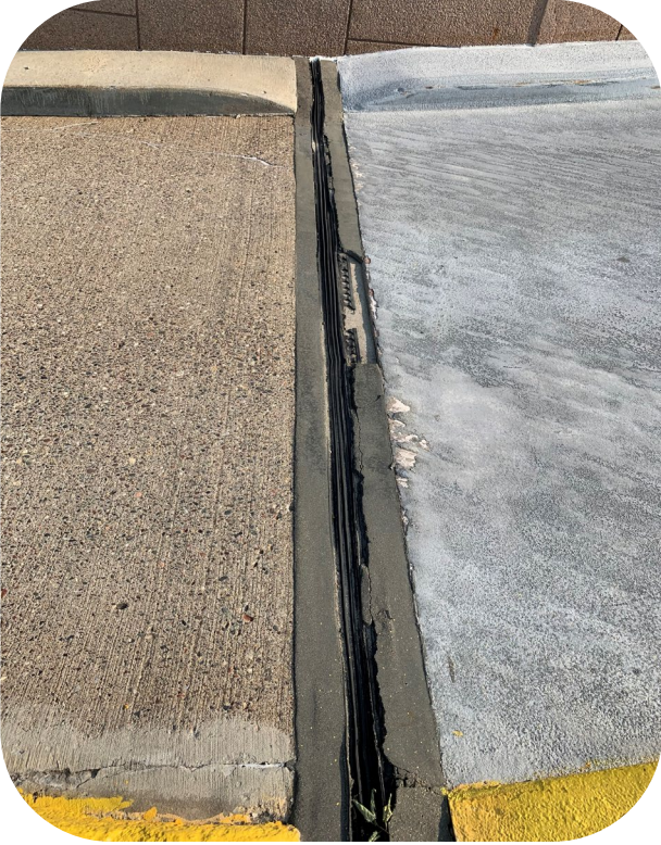
Typical Expansion Joint approx. $6,000 to replace
