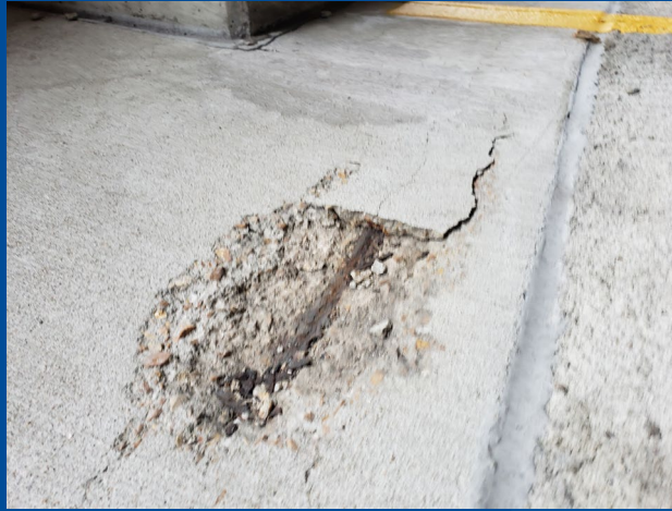
Reinforcement placed too close to the surface of the topping slab, resulting in the top surface failing due to rust jacking
