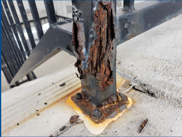
Failed handrail with rust jacking due to salts and weather
