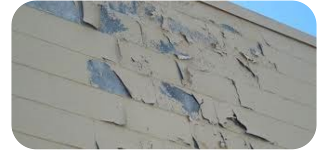
Delaminated Coating
