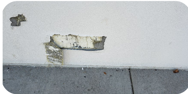
EIFS / Stucco Delamination
