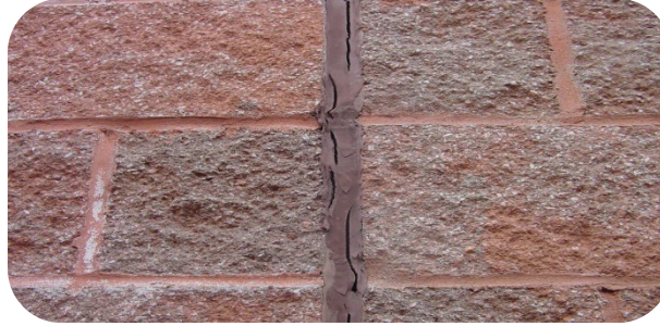
Sealant Failures
