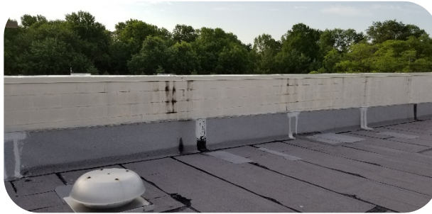
Roof Flashing
