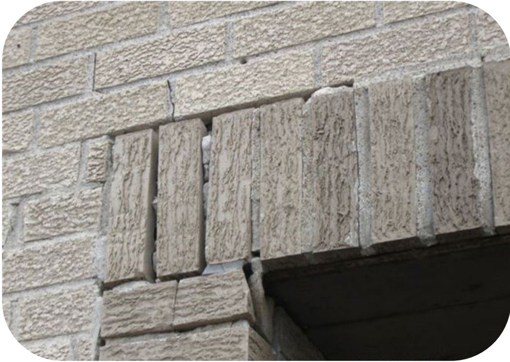
Deteriorated Mortar Joints
