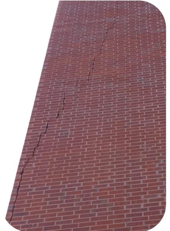
Cracking
