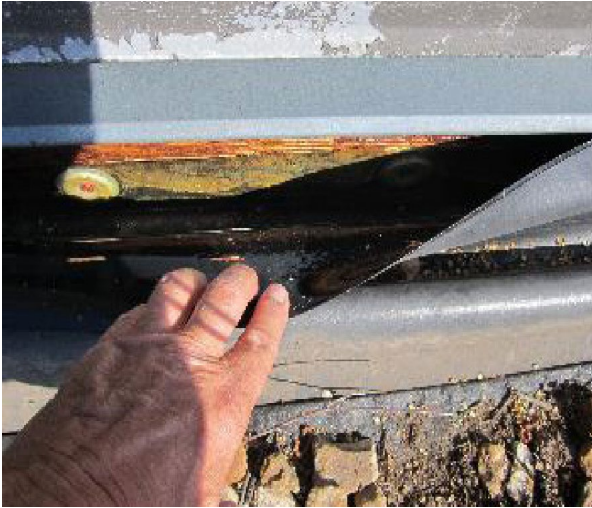
Failed Flashing
