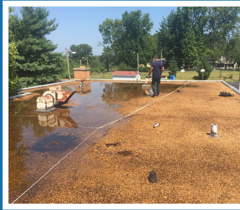
Clogged Roof Drains
