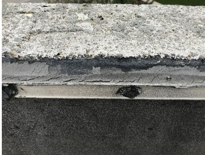
Failed Termination Bar Caulk
