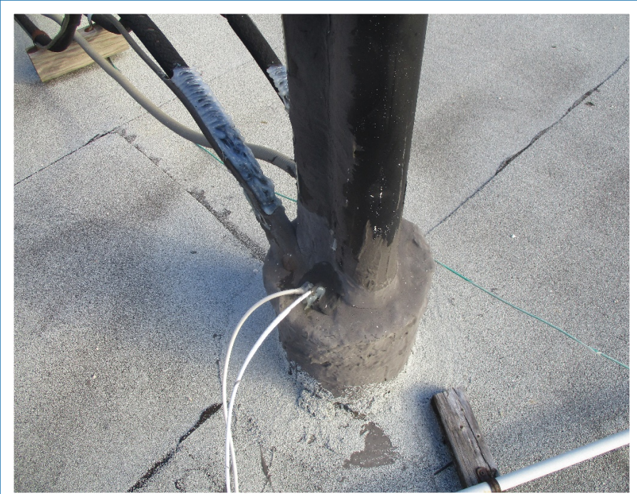
Improper Wire Flashing
