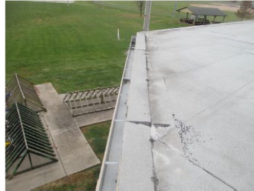
Photo 3: Overview photo showing the perimeter gutter observed to be performing properly.
