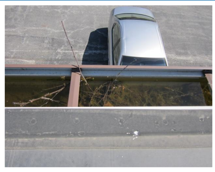
Debris Build-up in the gutter
