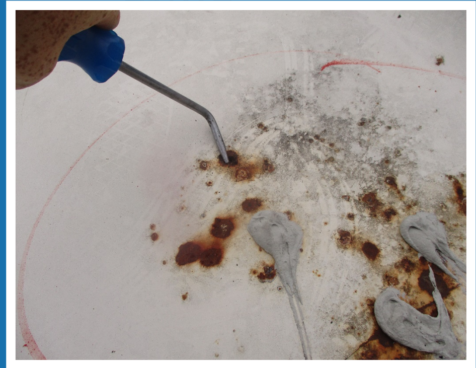
Holes Because of Rusted Coping
