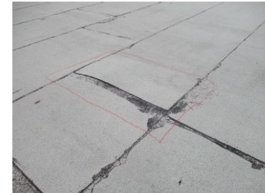
Photo 6: Additional photo showing a blister in the field of Roof 1 that has been marked for repairs.
