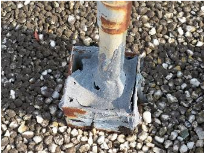
Deteriorated Pitch Pocket
