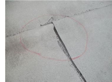
Photo 5: Photo showing a blister in the field of Roof 1 that has been marked for repairs.
