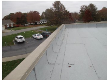
Photo 4: Overview photo showing the perimeter metal coping and flashings observed to be performing properly.
